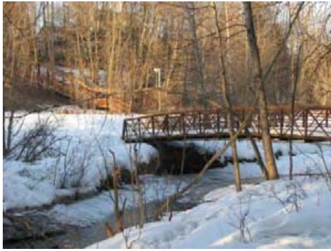
Bunker Street Bridge – east access from Chester Creek Trail
