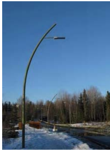
New Spenard Pedestrian Bridge West Access from Chester Creek Trail
